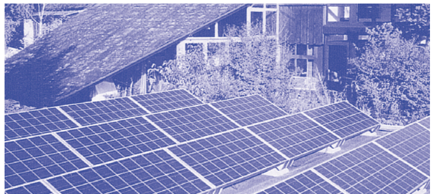
Photovoltaikanlage in Weinfelden
